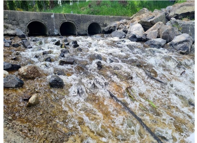
Fig 3. The Brooklands Road under high flows following the construction of the rock ramp.
