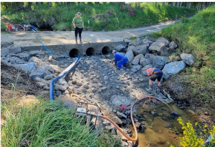
Fig 2. Construction of the Brooklands Road rock ramp, showing the low gradient ramps with rocks placed to reduce water velocity and provide resting areas for fish.
