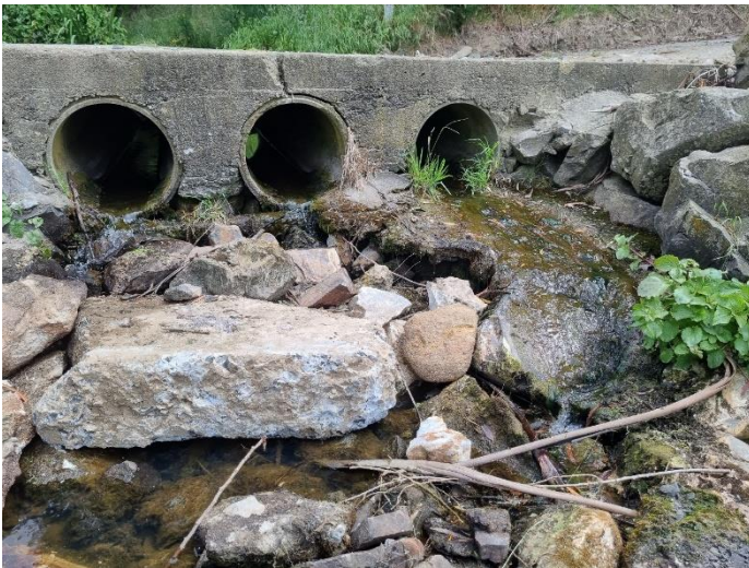
Fig 1. Downstream view of the Brooklands Road ford, showing poor fish passage characteristics present before construction of the rock ramp.
